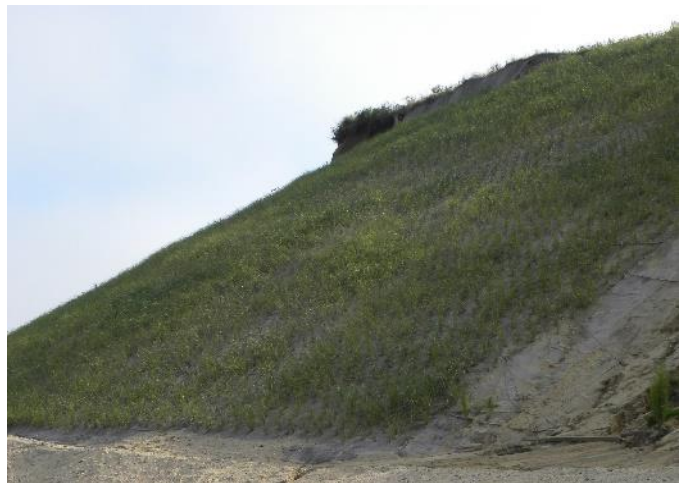
We propose to re-vegetate the eroded bluff face, like in this segment planted one year ago.
