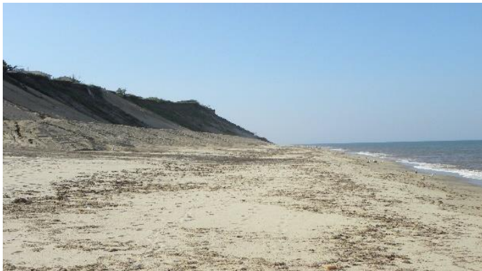
Wide beach in front of geotubes
