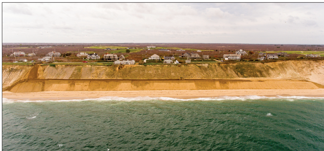
Geotubes covered by a sand template currently protect Baxter Road and homes along 950 feet of shoreline.
